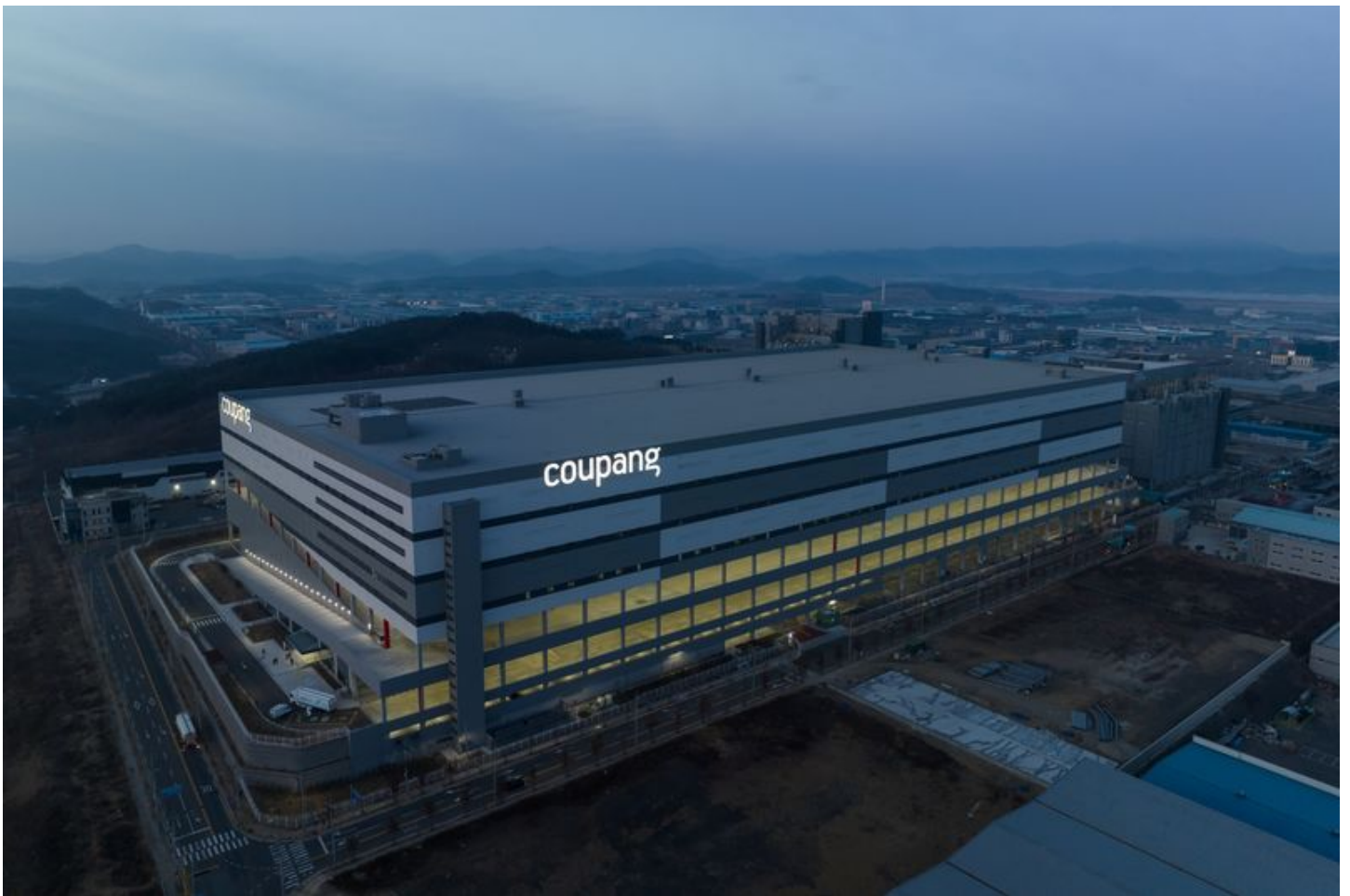
Coupang's fulfillment center building in Daegu. Photographer: SeongJoon Cho/Bloomberg
